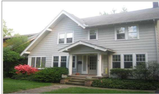
2822 Berkshire Road - View from Street
